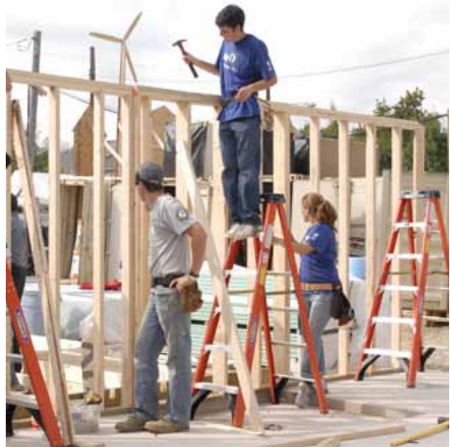
Shelter construction , Washington. D.C. USA. © UN-Habitat/Nathan Kihara
